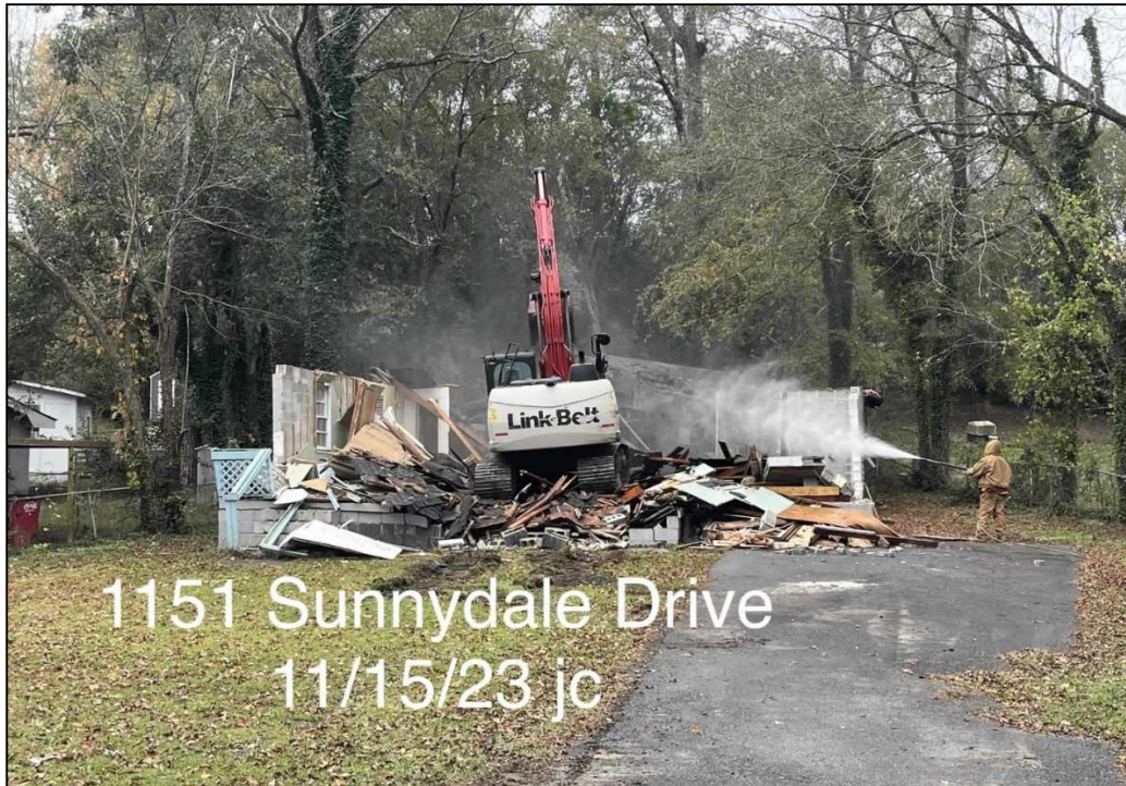
(1151 Sunnydale Drive mid-demolition; picture from Code Enforcement records)
